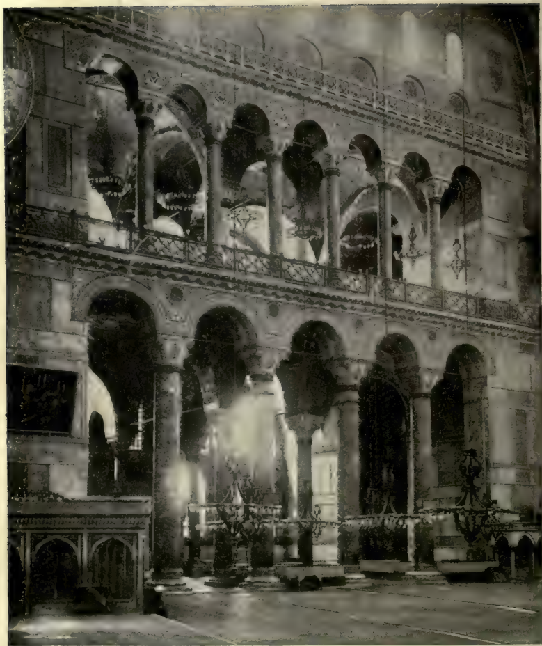
GROUND STORY AND GALLERY ARCADES FROM NAVE Santa Sophia, Constantinople
